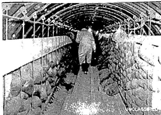
Tunnel interior with wooden rails for forklift and sandbag "benches" for utility lines and ventilation ducts. (U)
