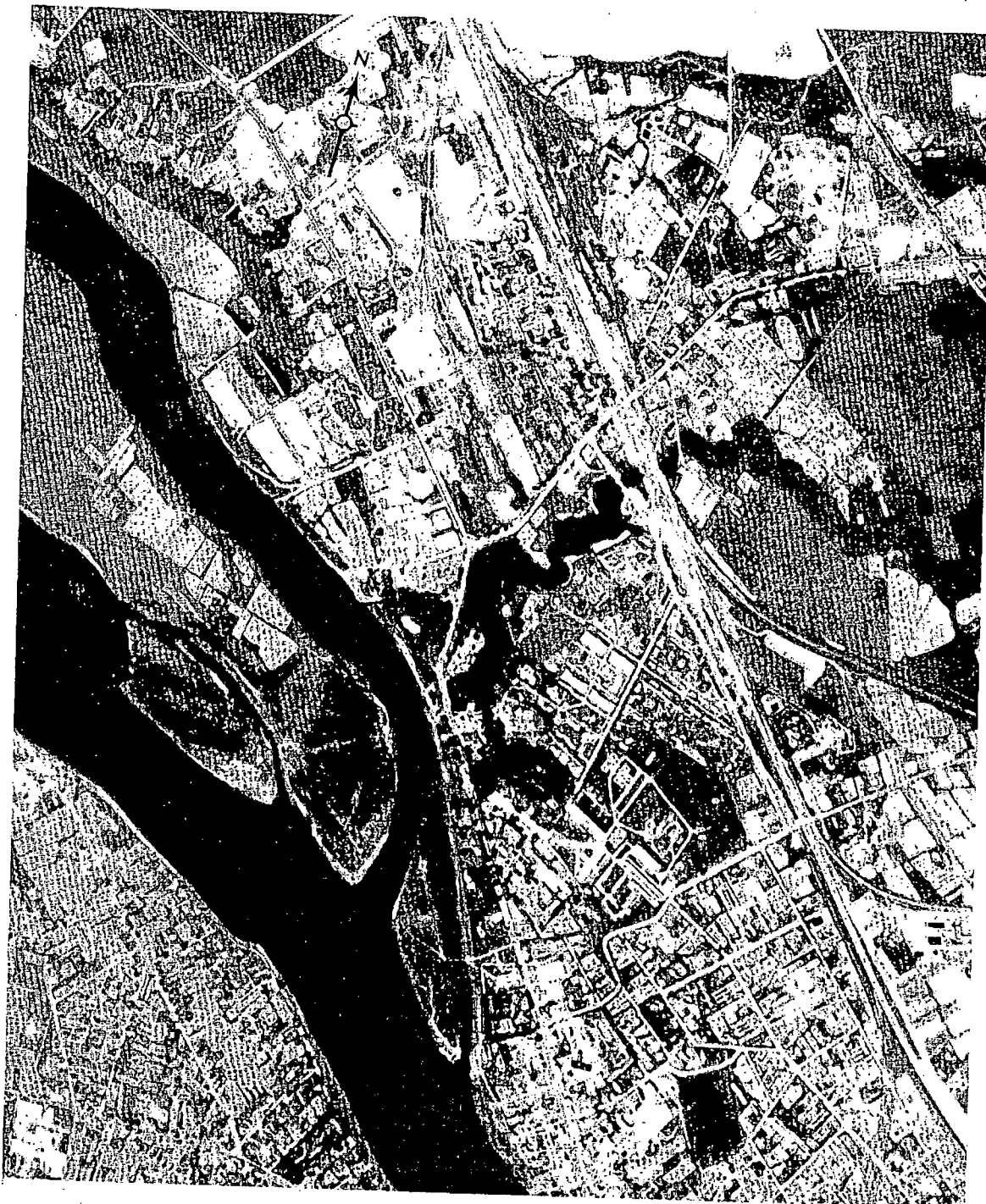
FIGURE 2. KRUSTPILS BARRACKS DVINA RIVER EAST, USSR, JUNE 1964.
