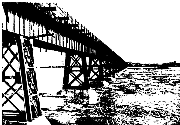
FIGURE 1. Railroad bridge over the Rud-e Karun at Ahvaz. The bridge rests upon the foundation of the great weir built by Shapur II in the fourth century A.D. (U/OU)
