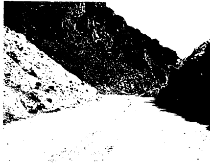
FIGURE 3. Eighteen-foot wide bituminous-treated highway, extending through a mountain pass 45 miles north of Ksar es Souk (C)
