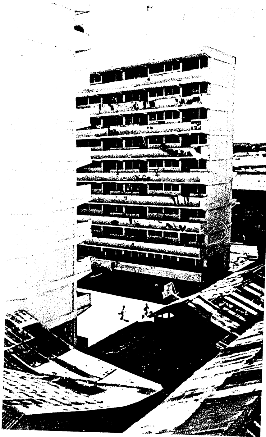
FIGURE 26. New apartments built in Panama City to replace slum dwellings (U/OU)
