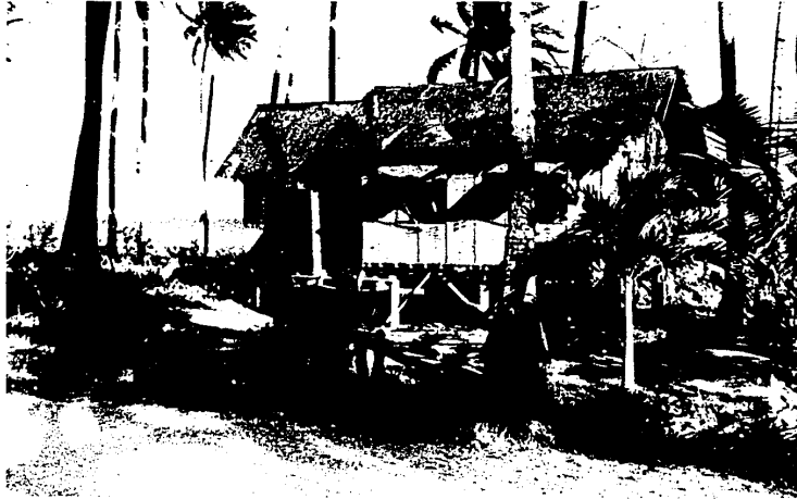
Typical peasant house along the coast of Negros Island. The dwelling has nipa walls and a thatched roof. (C)
