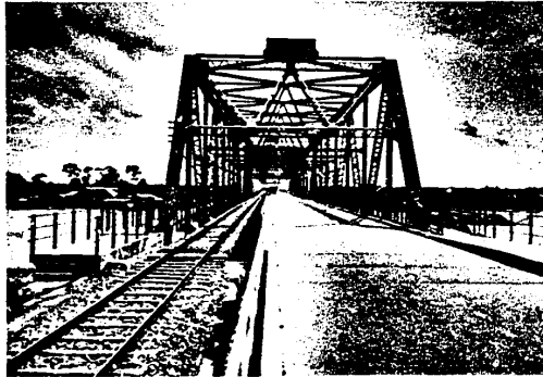
FIGURE 2. Rail-highway bridge over the Mae Nam Chao Phraya, 3.5 miles west of Bang Su. This 1,468-foot structure is the longest bridge on the RSR. (C)
