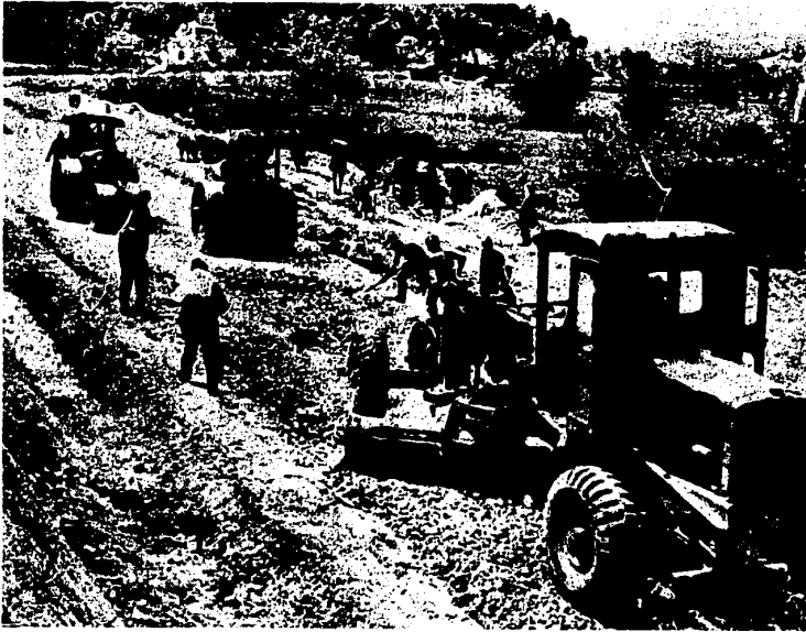
FIGURE 5. Yugoslav army engineers engaged in road construction (U/OU)
