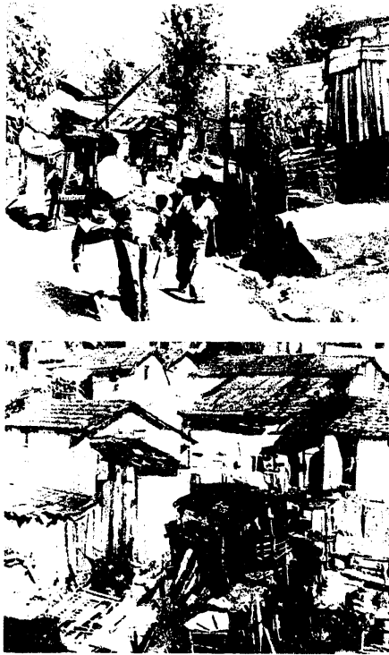
FIGURE 12. Improvised housing in Guatemala City. Tile, tin, and cardboard roofs cover dilapidated structures crowded together in narrow ravines and on steep hill-sides around the capital. (U/OU)
