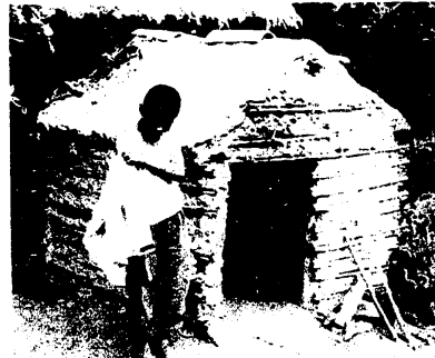
FIGURE 16. Temascal, or sweathouse. Water is poured over stones heated inside the adobe structure, creating a steam bath used both for bathing and for medical purposes. The door is covered with a blanket. (C)
