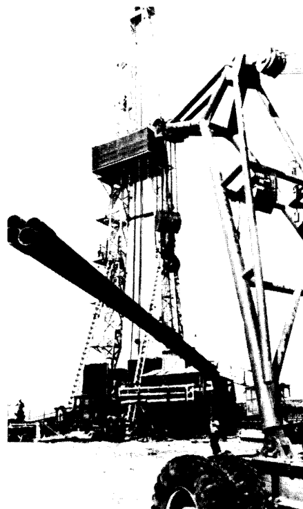
FIGURE 33. DRILLING RIG, NATURAL GAS WELL IN KALMYK A.S.S.R.
