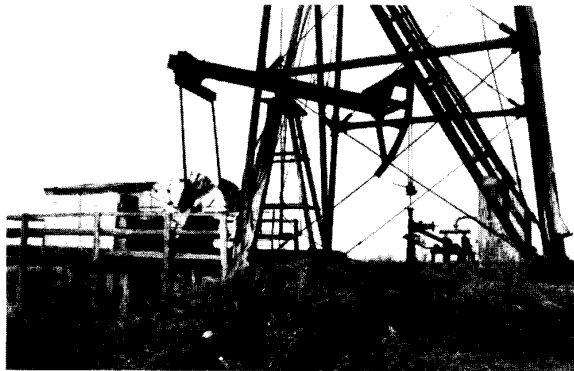
FIGURE 20. PUMPING OIL WELL AND WORK-OVER TOWER IN TUYMAZY OILFIELD
