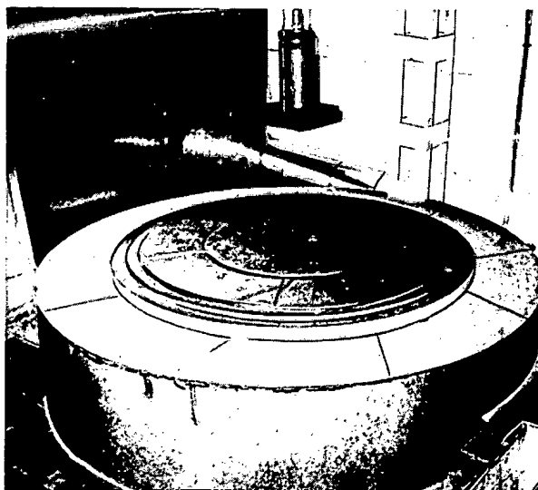
Fig. 2. External view of the shield and the operating surface of the RIZ stand reactor (top view).
