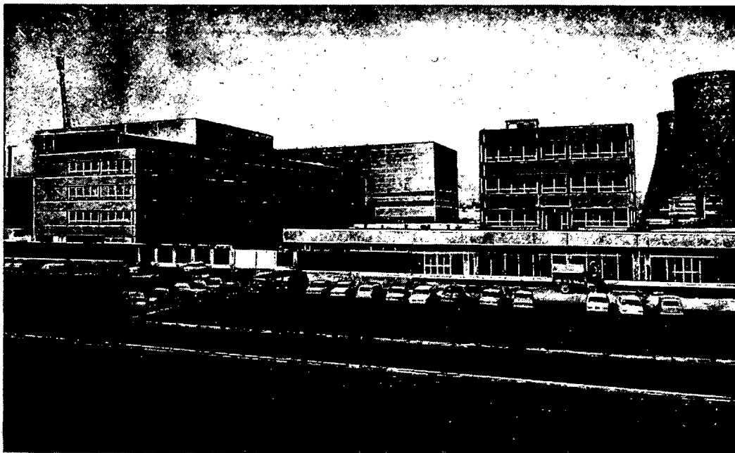
Fig. 2. General view of Armyansk nuclear power station.
