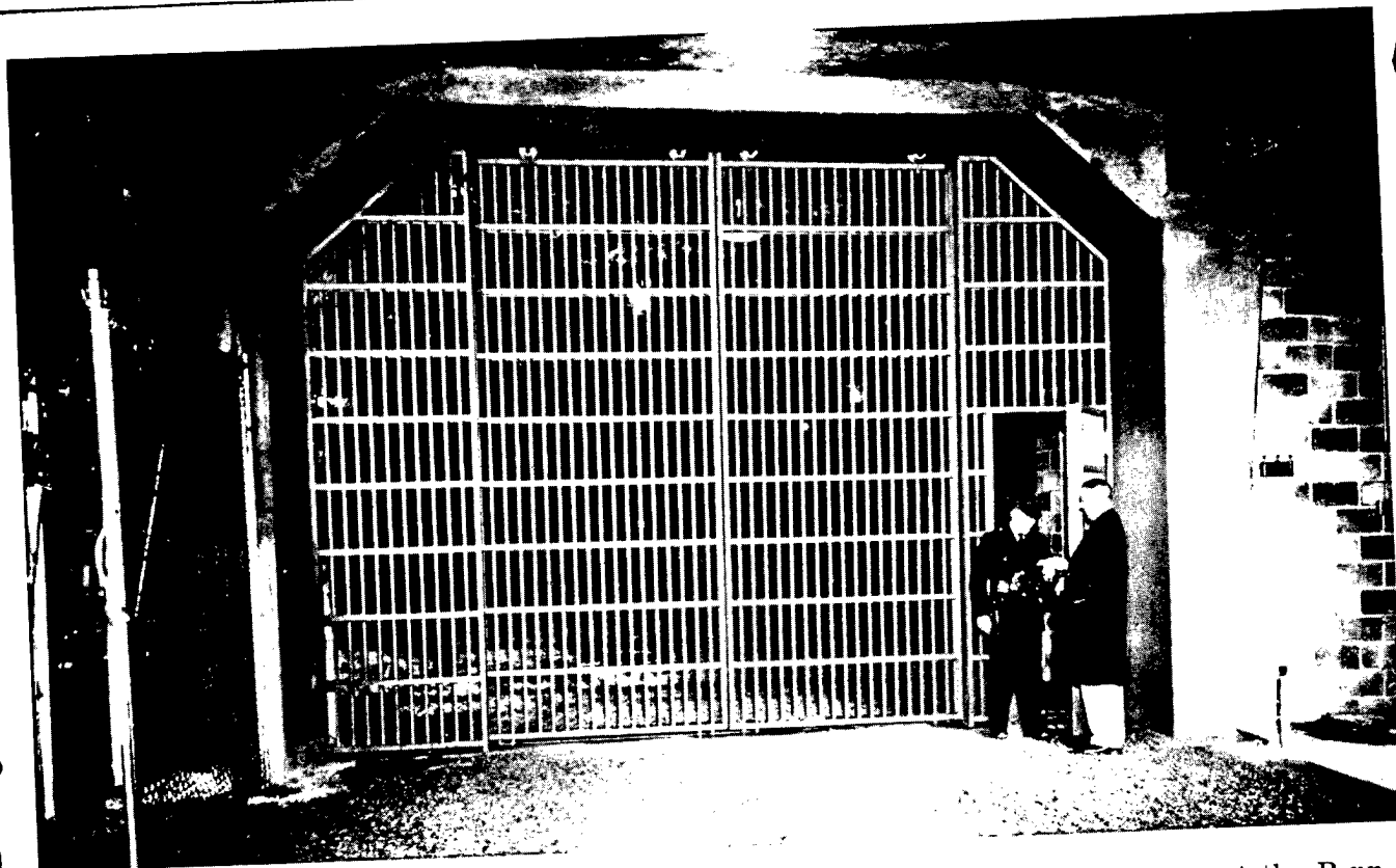
A three-ton steel portal gate and armed guards are part of the 24-hour protection at the Pennsylvania mine now being used by National City Bank for storage of duplicate records in the Bank's emergency operations program.
