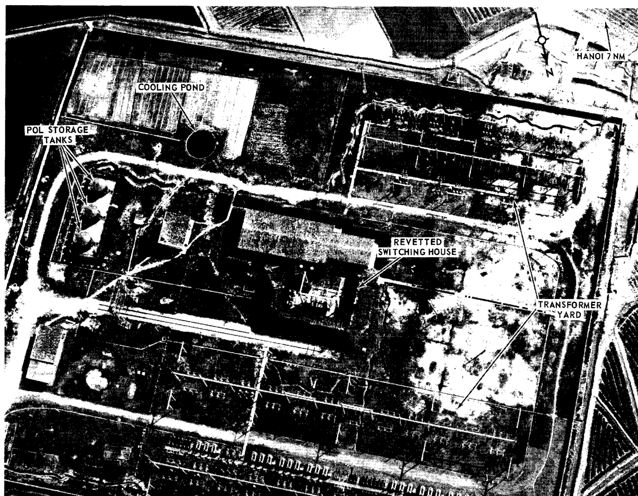
HANOI TRANSFORMER STATION LE PHAP, NORTH VIETNAM.
