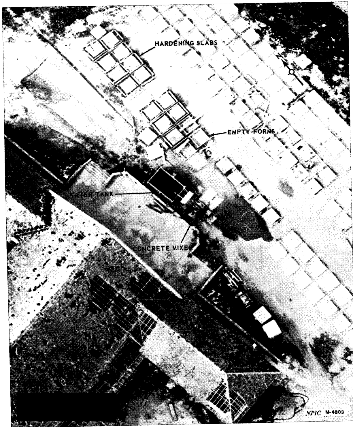
FIGURE 3. CONCRETE SLAB FABRICATION, PHUC YEN AREA.
