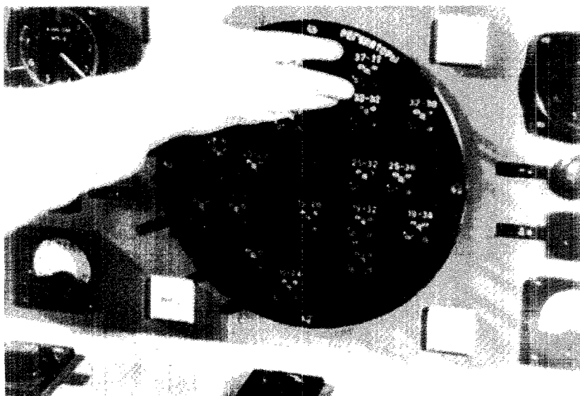
Figure 5a. Mechanism for regulating hoists of reactor control rods in 100,000 kw. atomic electric power station
