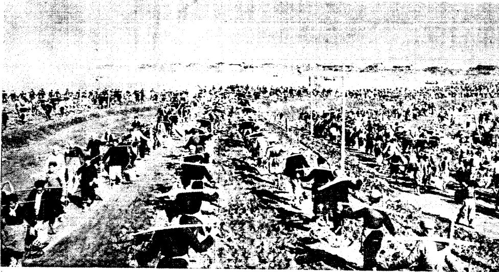
Dike construction at Tungting Lake in Hunan Province
