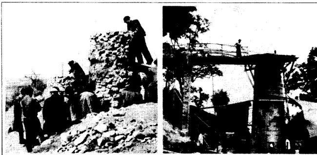
SMALL IRON SMELTING FURNACES IN SINKIANG AND SZECHWAN PROVINCES
