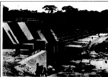
Hydroelectric Project on Djoue River near Brazzaville
