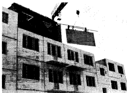
Large panel concrete structures such as this Soviet apartment house are to account for nearly two thirds of all state-built housing by 1965. [redacted]
