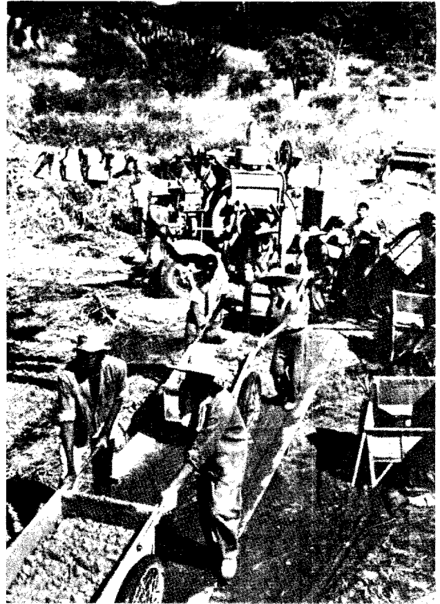
Local and Chinese personnel work on Tan-Zam Railroad.
