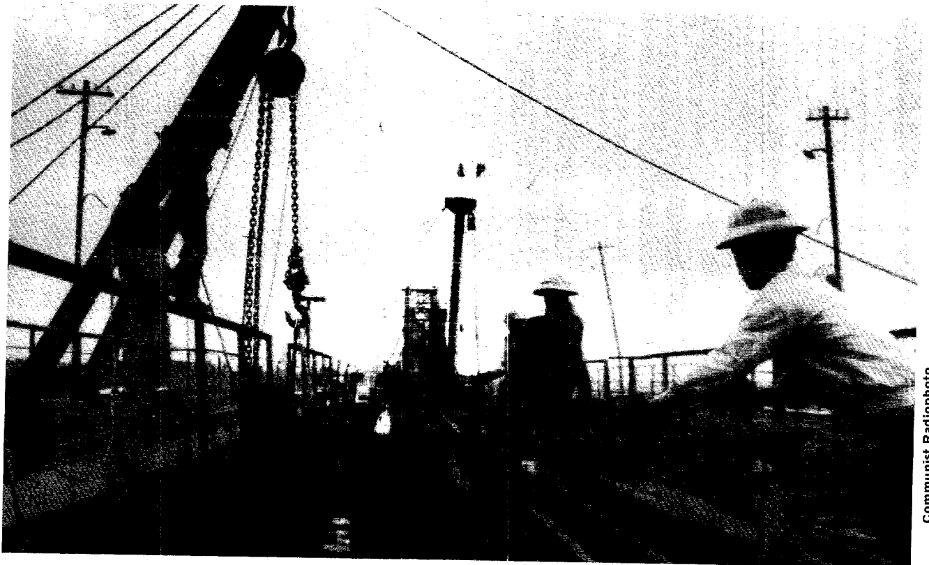
Repairing the Long Bien bridge
