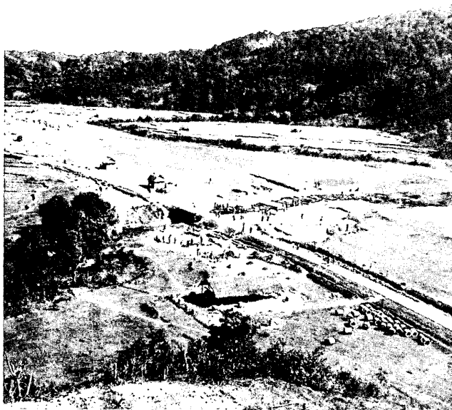
Figure 3. This airstrip under construction in a narrow valley outside the town of Sam Neua will accommodate C-47 type transport planes.
