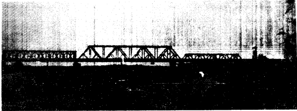
FIGURE 4. RAILROAD BRIDGE OVER THE ODER RIVER NEAR PODEJUCH, EAST GERMANY (July 1953). The span on the left is a 56-meter-long through truss of Roth-Waagner military bridging material bolted together by the Germans during World War II which has not yet been replaced by a permanent riveted span.
