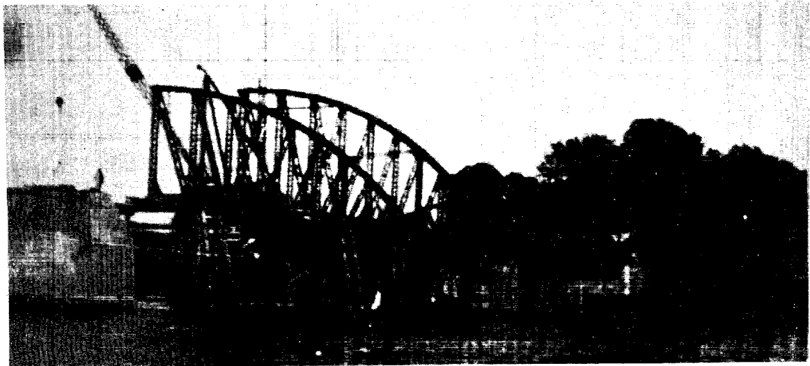
FIGURE 5. RAILROAD BRIDGE REPAIRS IN EAST GERMANY (July 1953). This railroad bridge over the Oder River near Kruenig was not replaced for 8 years following its destruction during World War II.
