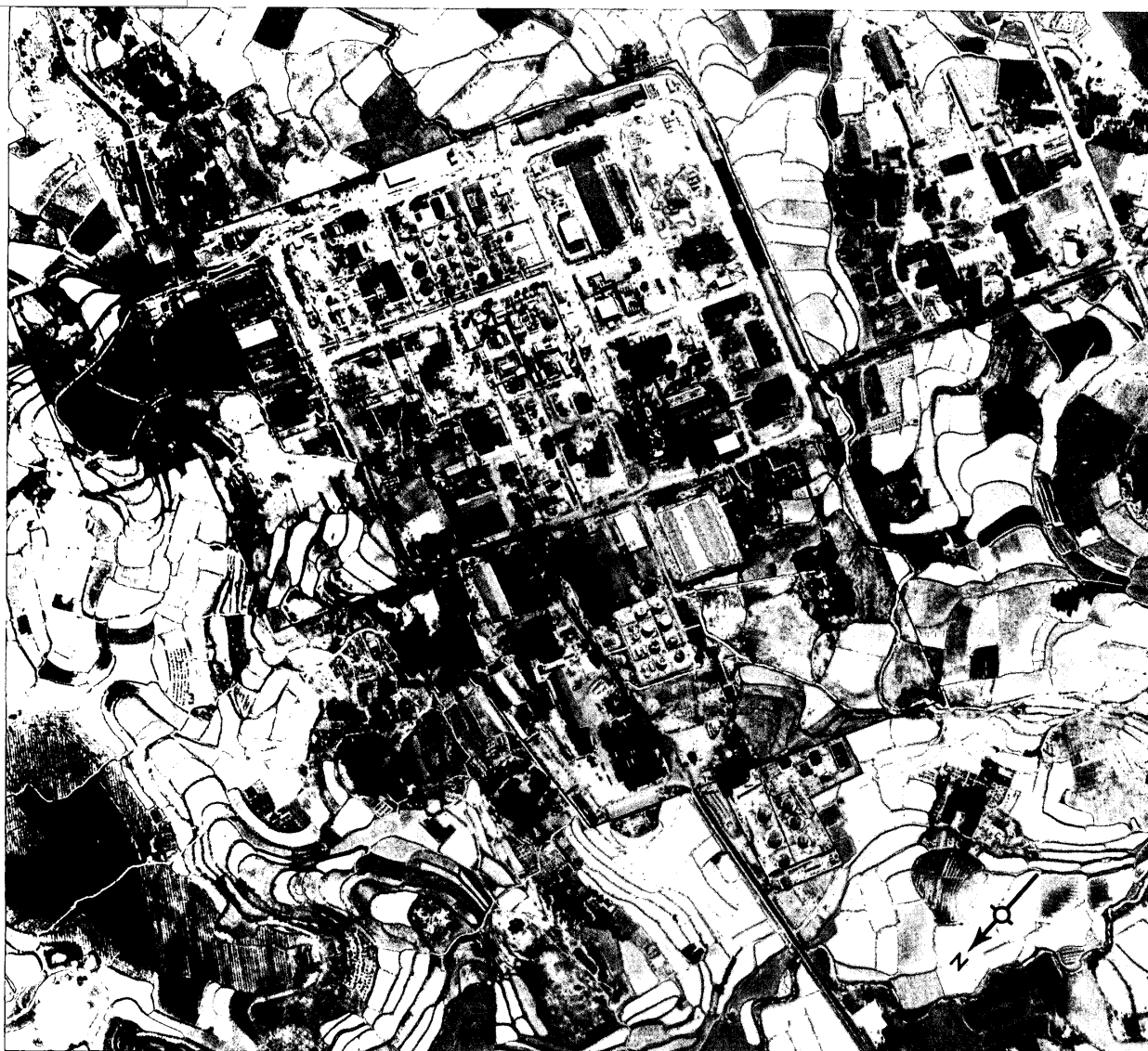
FIGURE 2. NAN-CHUNG PETROLEUM REFINERY
