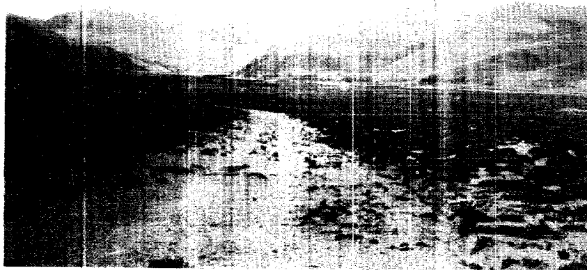
Figure 2. Part of the road between Khamba Dzong and Tingkye Dzong in southern Tibet. Open, flat valleys such as the one shown here are characteristic of much of Tibet, permitting roads to be built with little in the way of actual construction. This would be characterized as a "simple highway."
