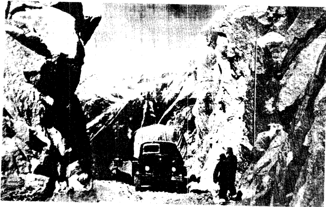
Figure 4. A section of the Szechwan-Lhasa road. The terrain of eastern Tibet is extremely rugged and mountainous. Rocky, north-south aligned ridges must be crossed by roads from Szechwan to Lhasa and southern Tibet. Construction is very difficult, costly, and time consuming.
