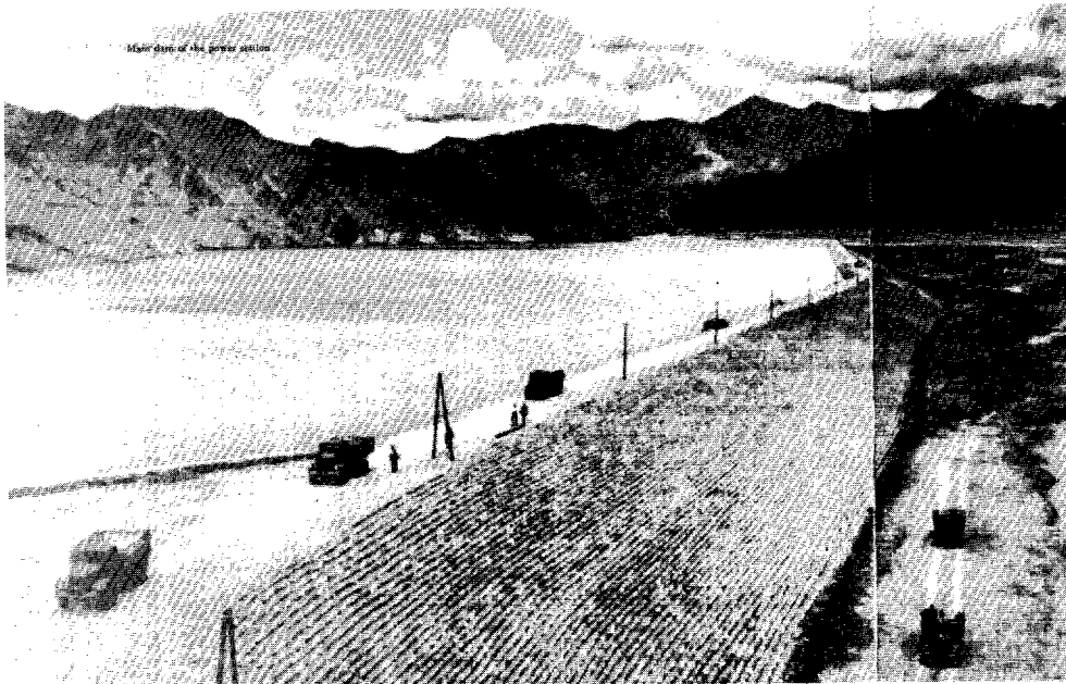
Figure 9. The dam near the Na-chin hydroelectric powerplant, built in 1960. This earthen dam east of Lhasa channels water from the Kyi Chhu to the powerplant, which presumably supplies Lhasa and its environs with electric power.
