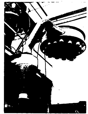
Filter units of a grinding mill.
