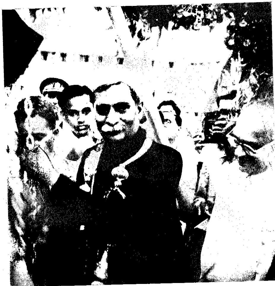
Dr. Rajendra Prasad, President, The Republic of India and Visitor, Indian Institute of Science, laying the foundation Stone of the Civil and Hydraulic Engineering laboratories.
