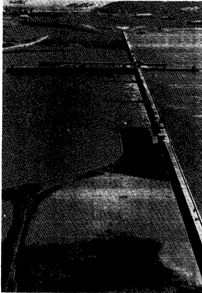
Figure 44. Jebel Aulia Dam and Lock ( 15^{\circ}14'N-32^{\circ}29'E ) on the White Nile about 21 miles south of Khartoum ( 15^{\circ}36'N-32^{\circ}32'E ).
