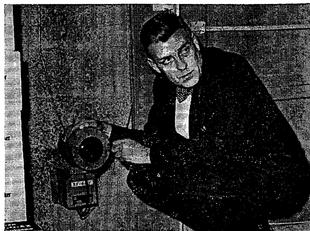
Security Chief checks alignment of Photo-Electric projector.
