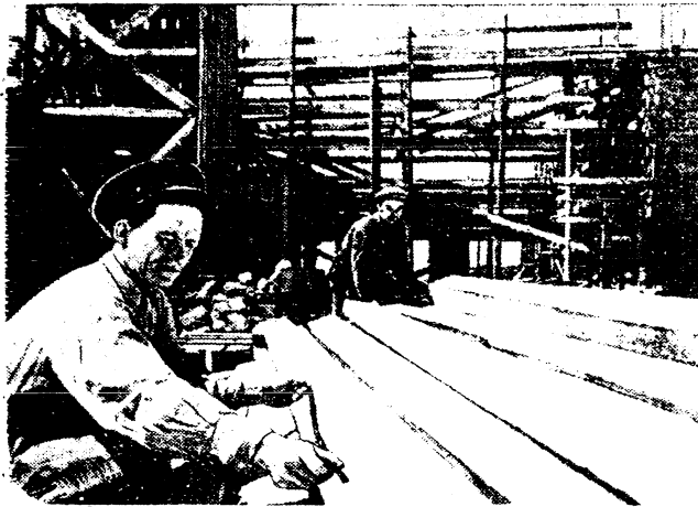
Fig. 15 - Preparing lumber for the roof of the new enginehouse at Adler station.
