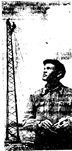
Fig. 35 - View of a contact tower at Nazyvayevskaya station.
