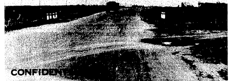
FIG 5. View of the newly-constructed section of the Brest-Moscow highway. Looking SW from a point 2 miles West of the interchange with the Minsk-Slutsk highway. (C)
