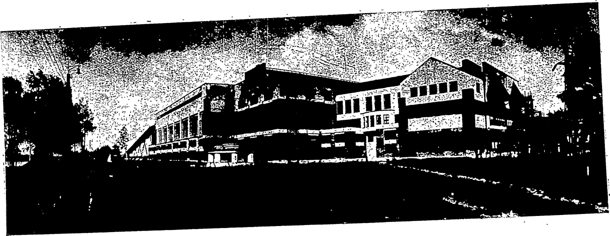
View from the turbine hall side.
