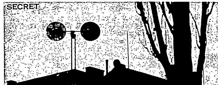
FIG 87. BUG EARS Microwave Radio Relay Antennas In A Fixed Installation. (U)
