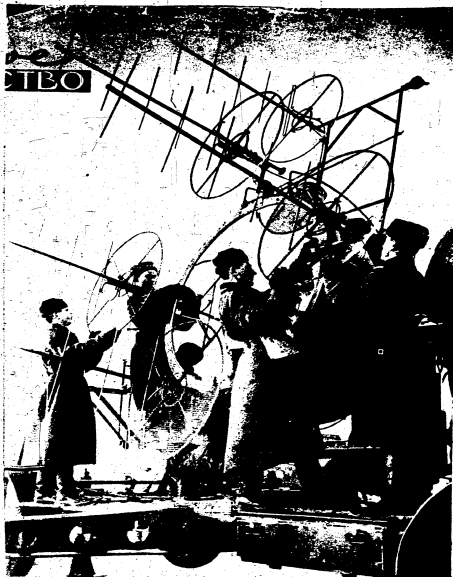
Fig. 69 - Searchlight-control radar in operation.
