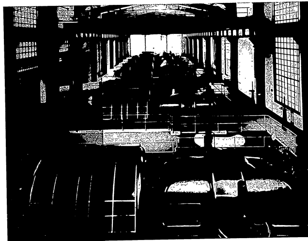
Power station with seven condensation turbines of 12.000 KW each. (SOCIETA' LARDERELLO - 1937).
