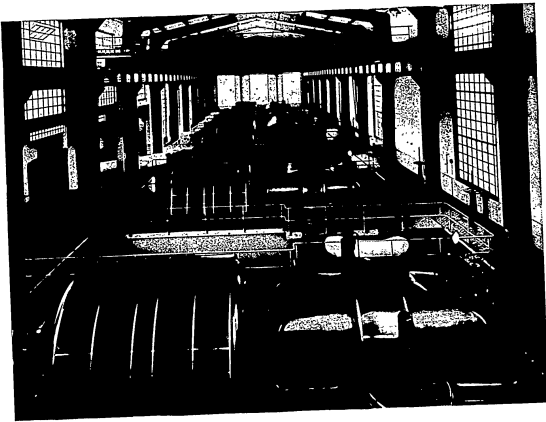
LARDERELLO N. 2 TURBINE ROOM WITH 7 TURBINE-GENERATORS OF 12,000 KW
