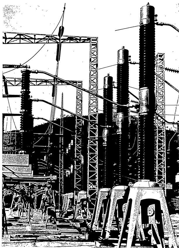
Fig. 18 - Type OGORD/OCERD 220 circuit breakers and isolating switches for 220 kV installed in an outdoor substation in Central Italy.
