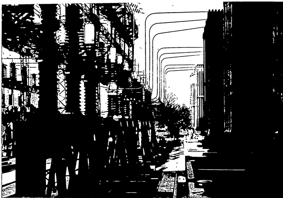
80 kV Outdoor sub-station equipped with «Galileo» Circuit Breakers
