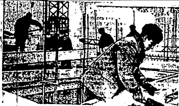
Fig. 53 - Building of Tomylovo traction substation Source: Oudok, 28 March 1957, p. 3
