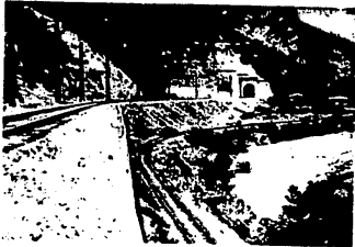
Fig. 45 - Newly constructed and electrified Zestafoni-Pereval run of the Zestafoni-Chistura line. In the lower right - an old narrow-gauge line.
