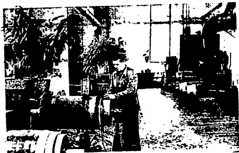
Fig. 51 - Machine shop for electric equipment at Perm' Enginehouse
