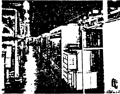
Photo 3. Klystrons and Their Pulsars Arranged in the Klystron Room
