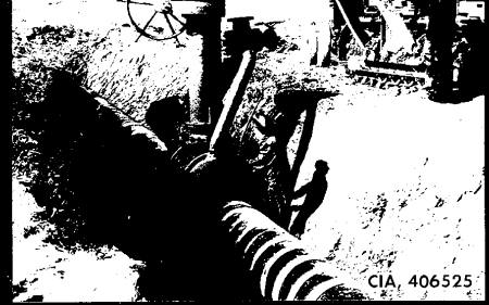
VALVE INSTALLATION
