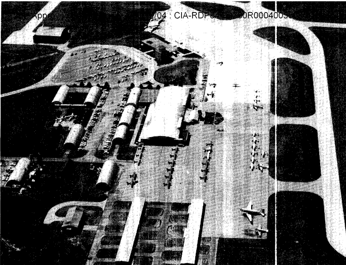
The Institute of Aviation operations center at the University of Illinois-Willard Airport. The University of Illinois has operated the Airport since 1946. The $4 million facility houses many of the research, public service, and educational activities in aviation of the Institute.
