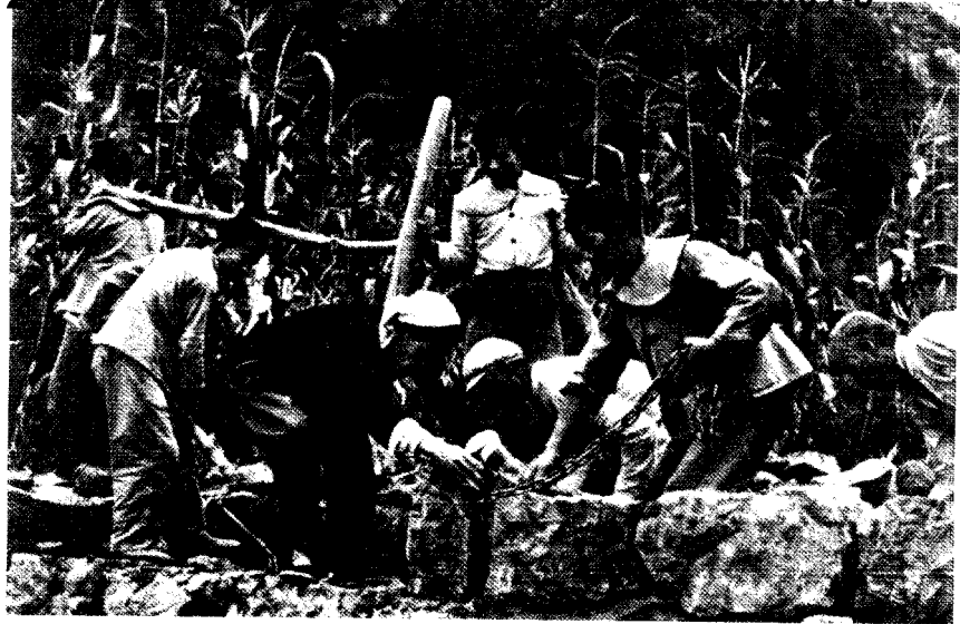
Figure 7. Transforming nature requires enormous amounts of labor. Building dry-wall stone terraces at Ta-chai; improving ordinary fields to high-yield fields by providing dependable supplies of water; elaborate earth-walled terraces to combat erosion in North China.
