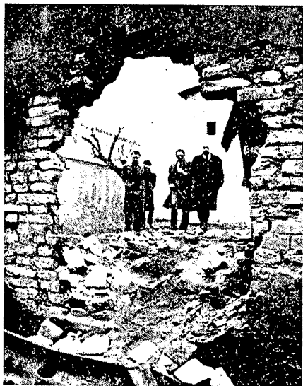
Police inspect blown-out prison wall
