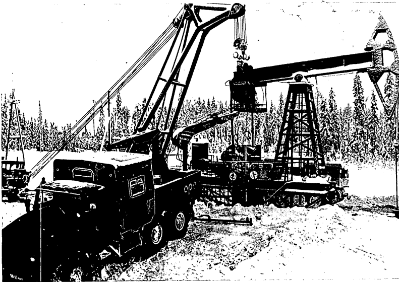
Periodic servicing is required to maintain mechanical sucker rod or beam pumping units.
