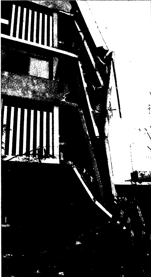
Figure 2. Structural damage due to earthquake.
