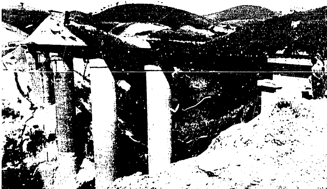
Bridges on the Mlimba-Makumbako section to the Tan-Zam Railroad.
