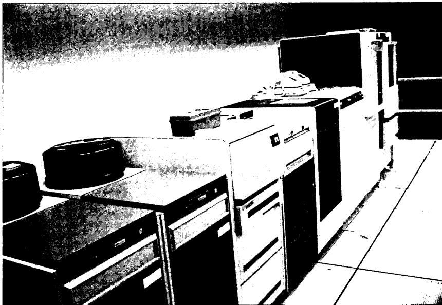
FIGURE 4-17. EICC COMPUTER ROOM
