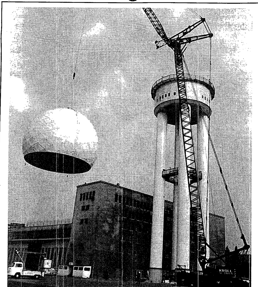
New radar system at Tempelhof Central Airport, Berlin, will be housed in 53-ft.-dia. radome shown as it was installed atop a 233-ft. tower at the airport. The system will employ an enhanced version of the AN/FPS-117(V) radar developed for USAF's Seek Igloo program and an automation/display system with four-color controller consoles.
