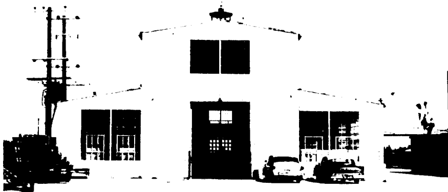
Missile Assembly Bldg
