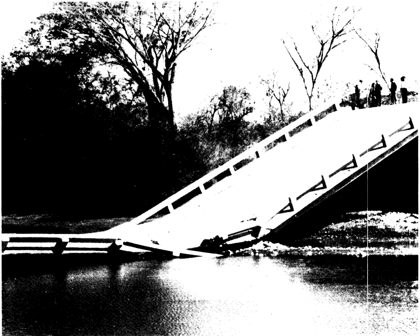
Bridge over the Rio Negro, destroyed on March 14, 1982 by ex-Somocista National Guardsmen.
