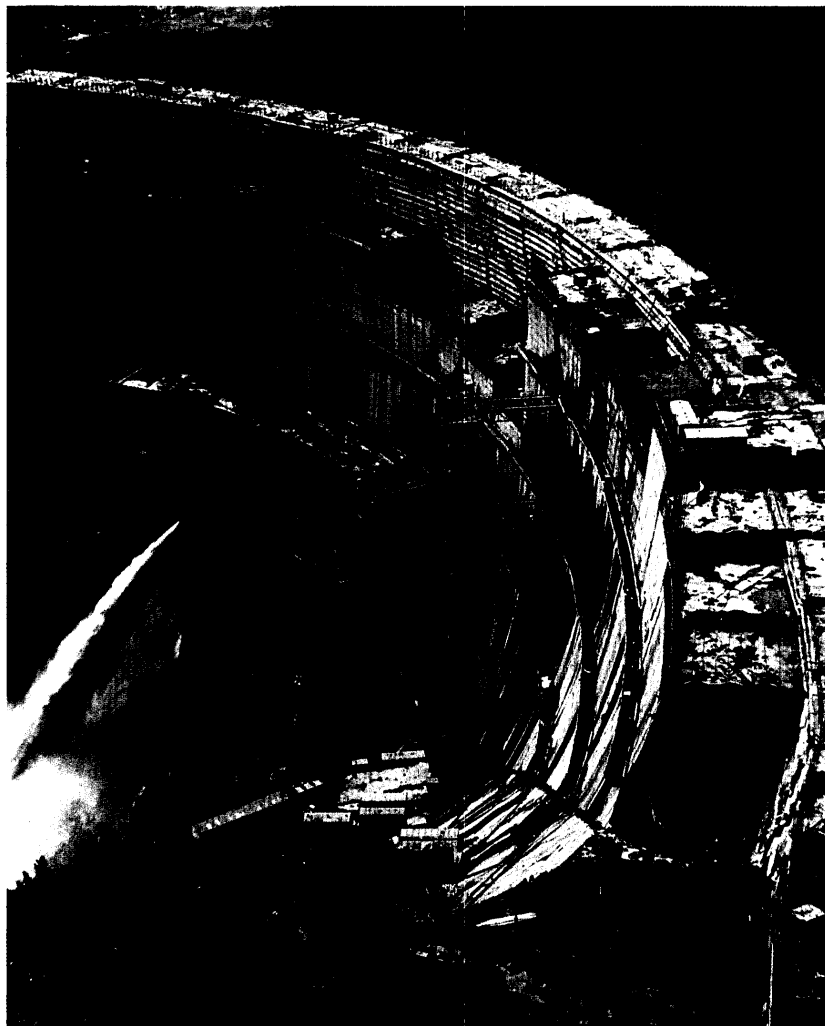
Construction of 1,325-MW Inguri Hydropower Dam across Inguri River in the Caucasus Mountains, Georgian SSR.
