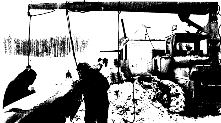
Pipe is welded at storage area welding bases along the pipeline by crews using either manual arc techniques or semiautomatic units.
