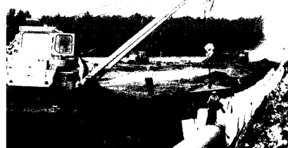
Concrete blocks are used in areas of swamp and permafrost to support the pipeline.
