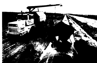
Pipe sections being welded by manual, arc-welding technique.
